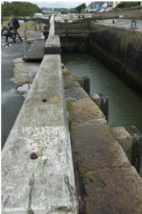
Close up of the dislodged gate on the Sea Lock
