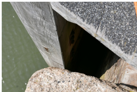
This is the gap which appeared due to the problem with one of the outer gates on the Sea Lock
