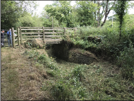
Photo 8 - Gadlock Bridge almost cleared
