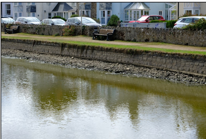
The low water level along the bank on Breakwater Road
