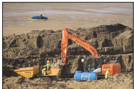
Work underway on Tommy's Pit
