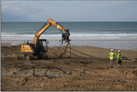
Removing cables from Crooklets Beach
