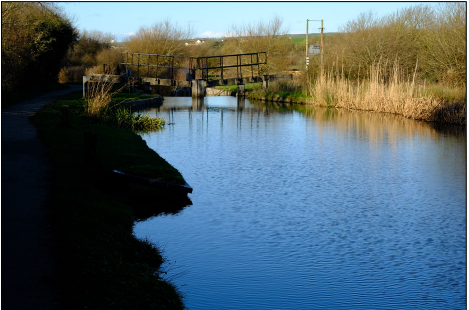
Dredged Upper Pound looking towards Whalesborough Lock
