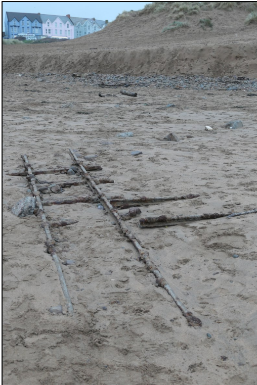
Remains of the Sand Railway uncovered on Summerleaze Beach at the end of December
