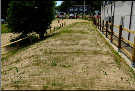
The flood embankment behind the TIC with the wild grass mixture now established
