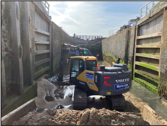
Dredging the Sea Lock (left and below)
