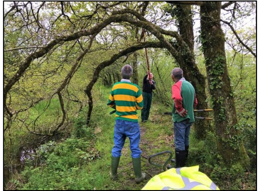
Overhanging tree being removed
