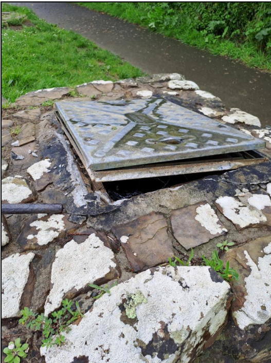
Damaged inspection pit cover
