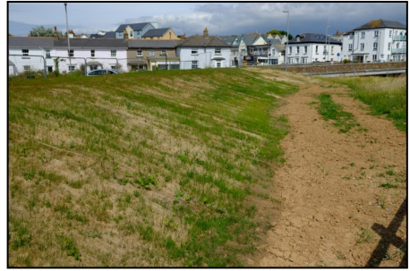
The flood embankment behind the TIC with the wild grass mixture now established
