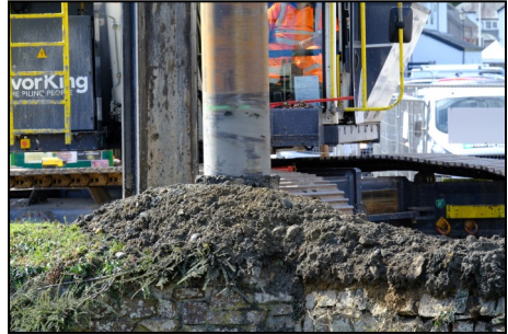
Close-up of drilling
