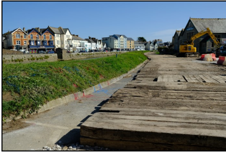
Decking to protect road surface
