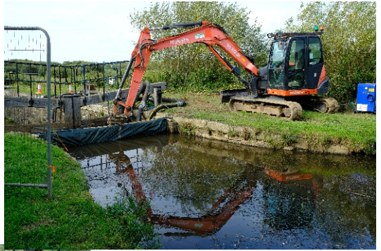
Positioning pipes to pump out from behind upper gates
