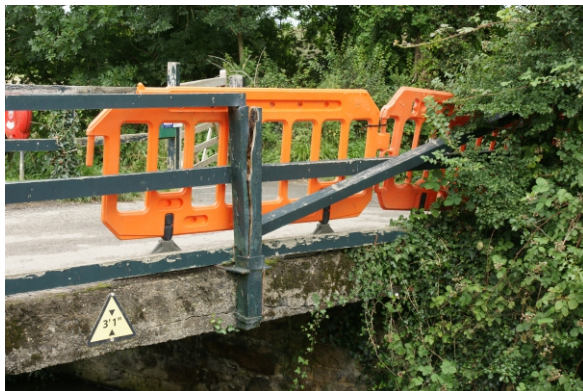
Damaged rails on Rodds Bridge
