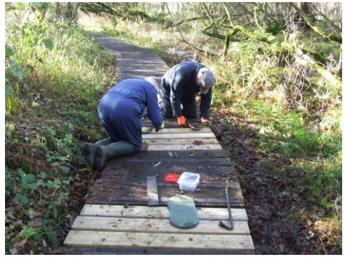
Nailing down the new boards
