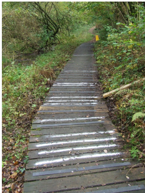
Marked replacement boards
