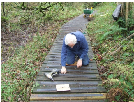
Fixing the non skid pads
