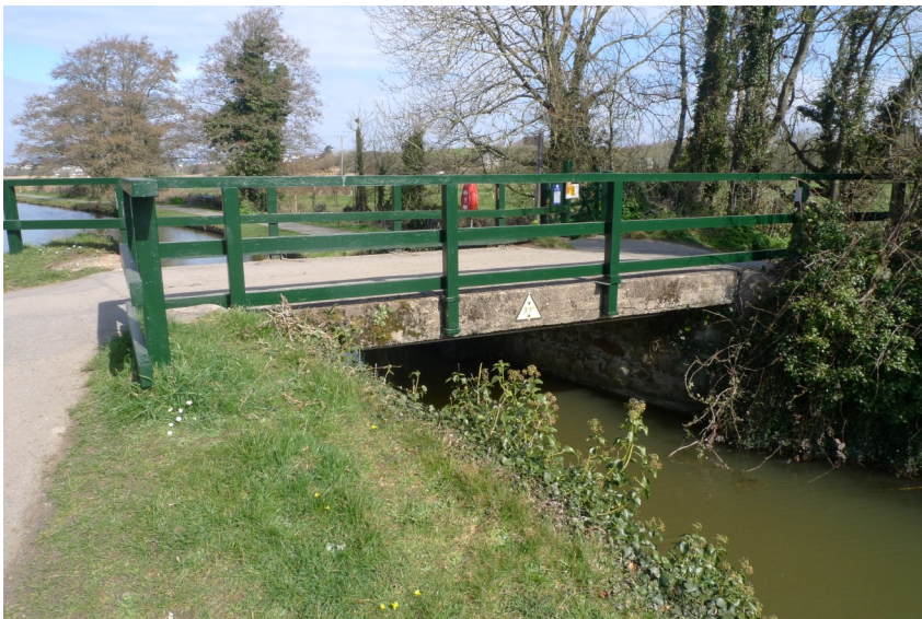
New rails installed at Rodds Bridge. The photo on page 21 of Tub Boat No.93 shows the damage
