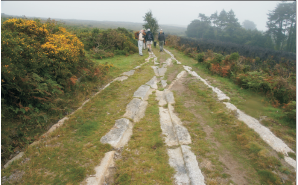
A fine view of the granite tramway showing a junction. Photo: M. Moore
